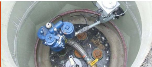
Owners and operators of federally regulated UST systems must have a release detection method, or combination of methods for connected underground piping that routinely contains product.
